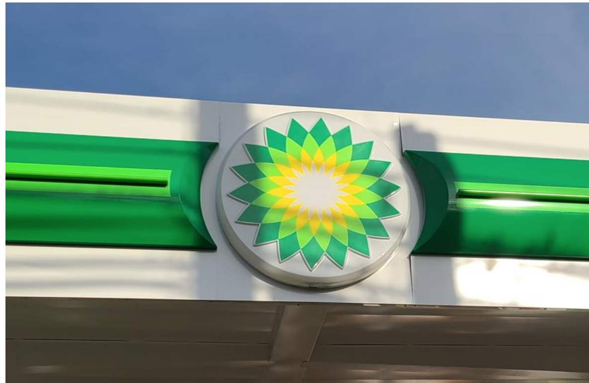
Figure 4: Example of a refaced BP fuel pump canopy with a 3-D fascia band.
